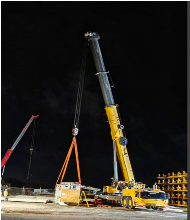
Night lift of a transformer into final position at the substation.
