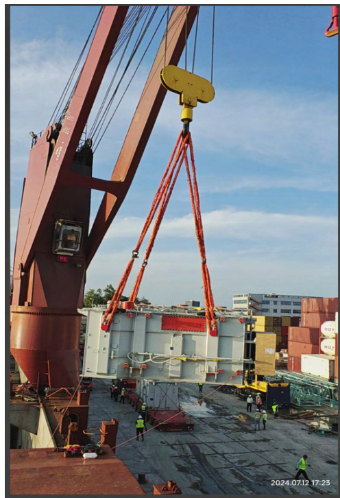
Ship-mounted crane lifting a transformer unit directly from the vessel at the port of Georgetown.
