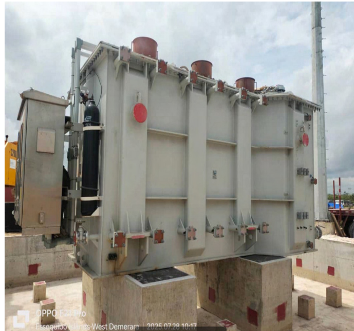
A transformer in its final position on the substation foundation.
