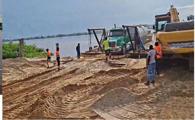
Excavator support preparing the sand ramp for barge loading.
