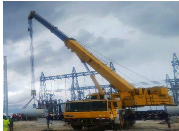
Tandem mobile cranes positioning a transformer at the substation.
