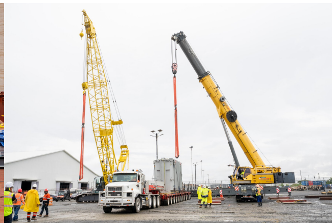
Two mobile cranes performing a synchronized tandem lift at the JFL warehouse facility.
