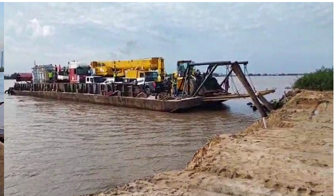
The barge underway across the river with cranes and support vehicles aboard.
