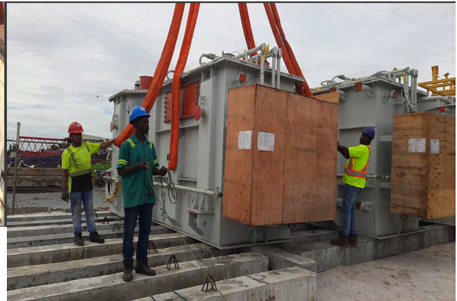
Crew rigging a transformer for lift-off at the foundation site.
