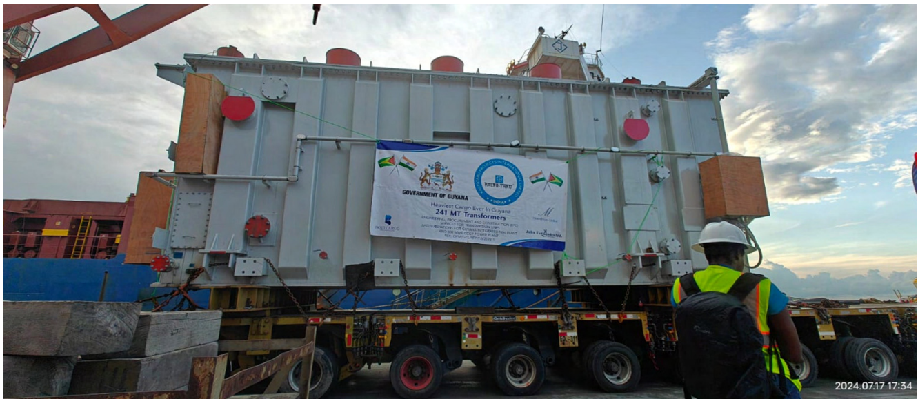
The 241 MT transformer, the heaviest single piece of cargo ever recorded in Guyana, staged on a multi-axle trailer at the port.
