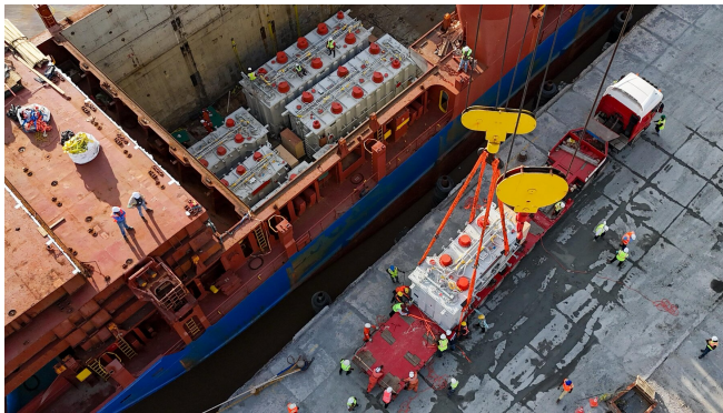
Aerial view of a transformer being lifted directly from the vessel's hold onto the quay.
