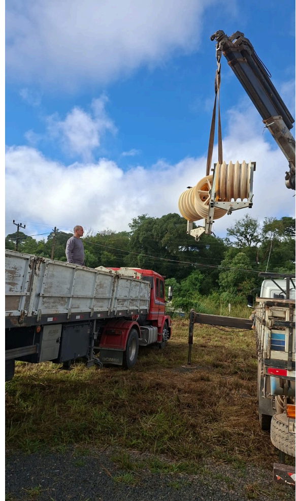
Crane-assisted handling of cable equipment at the project site.
