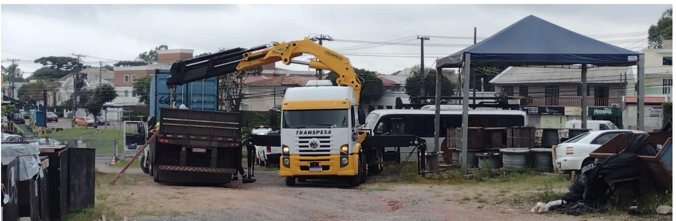
Crane-equipped vehicles coordinated at the operating yard.
