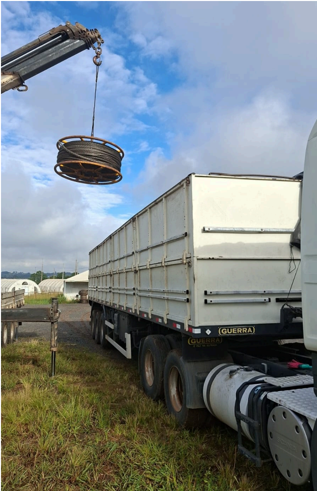
Crane-assisted transfer of a wire-rope reel.
